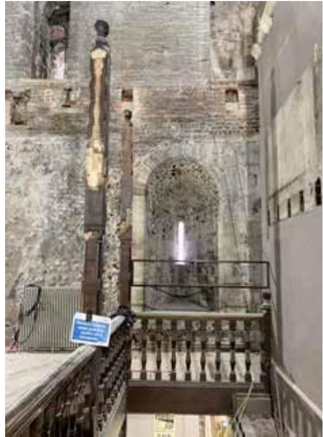
Fig 19 Southwest corner of the keep, with staircase salvaged from the site
