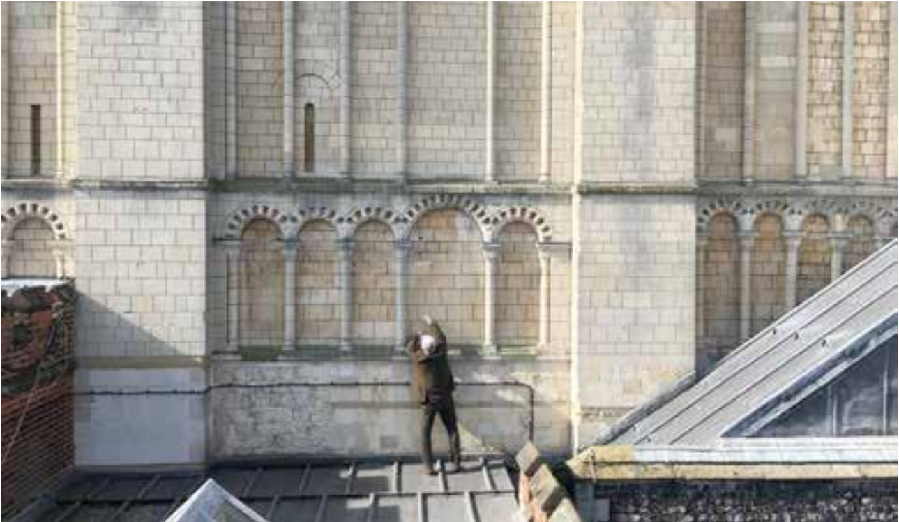
Fig 16 Anomalous arch in the external arcading of the east wall of the keep
