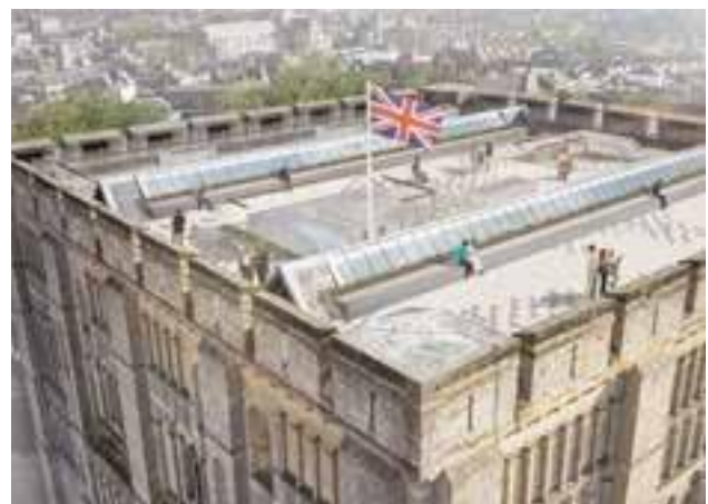
Fig 7 Accessible roof terrace with retained crenellation
