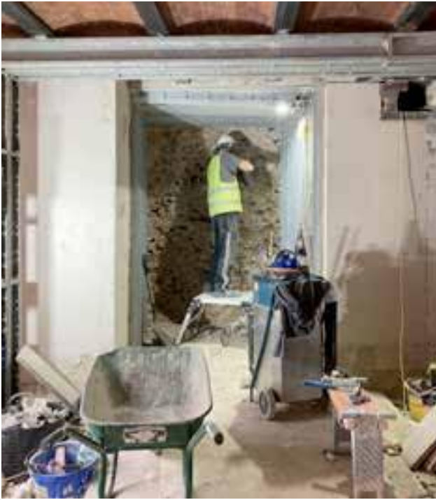
Fig 13 Opening through the north wall from outside
