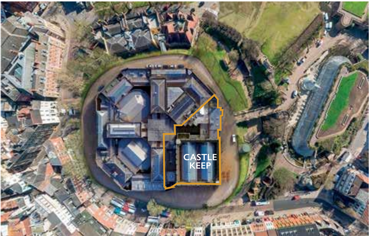
Fig 2 Birdseye view showing the extent of the project site, north to the left
