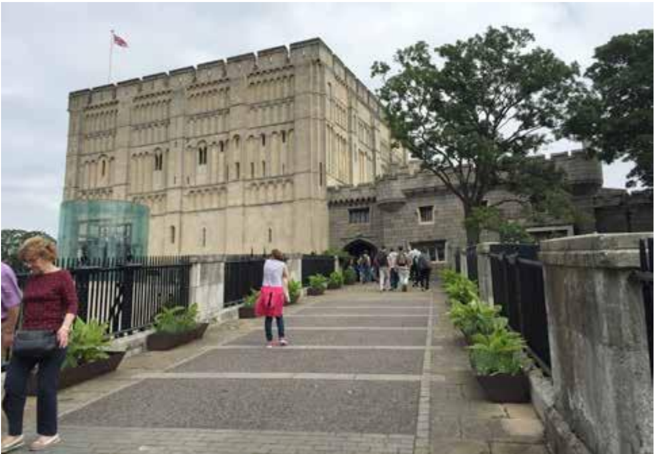
Fig 1 Norwich Castle keep with the existing William Wilkins building to the right
