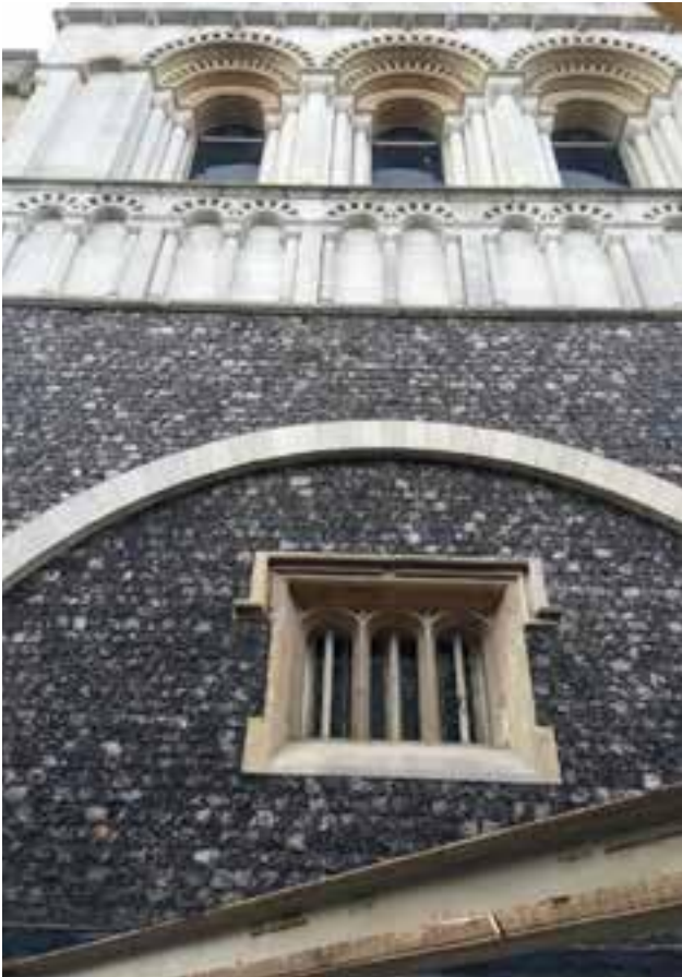
Fig 18 Flintwork wall to the Bigod Tower
