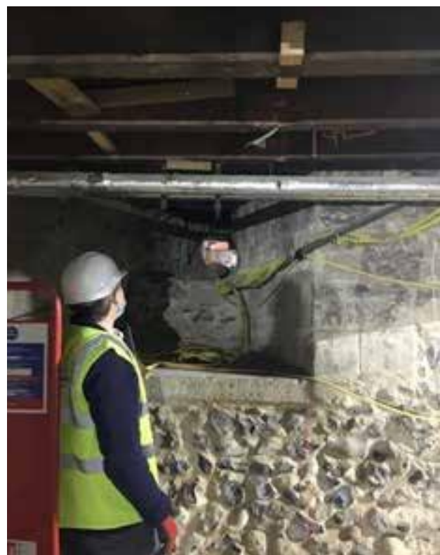
Fig 12 Norman cill and jambs to be preserved
