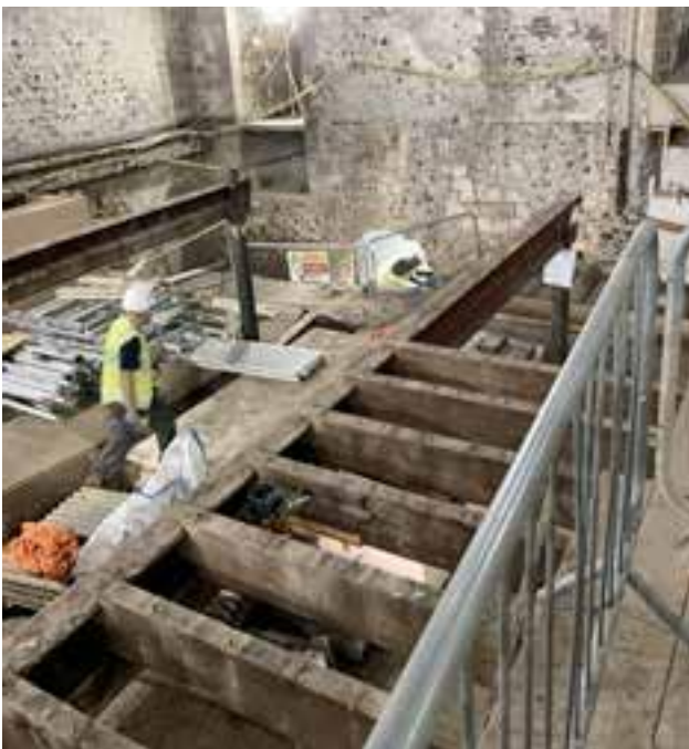
Fig 15 Inside the keep, new opening bottom centre
