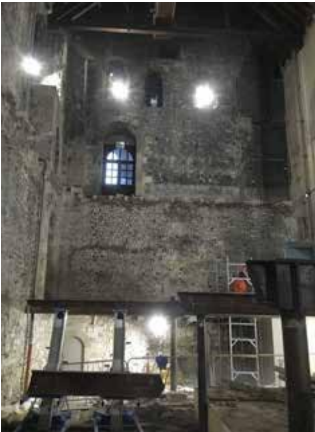
Fig 22 View of east wall highlighting the original volume of the spaces
