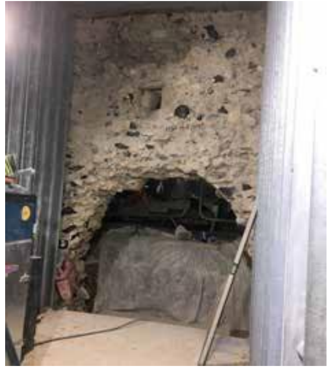
Fig 14 The new opening breaking into the keep
