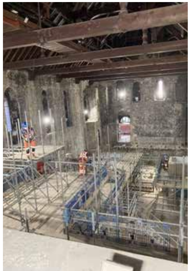
Fig 20 View looking east toward Norman door leading into the Bigod Tower
